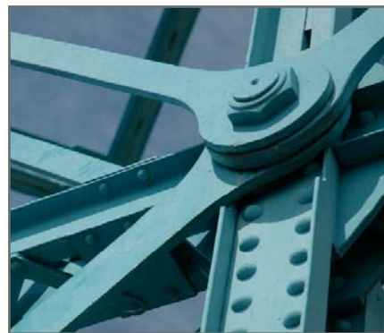
Structure analysis and monitoring, e.g. Civil Engineering.
